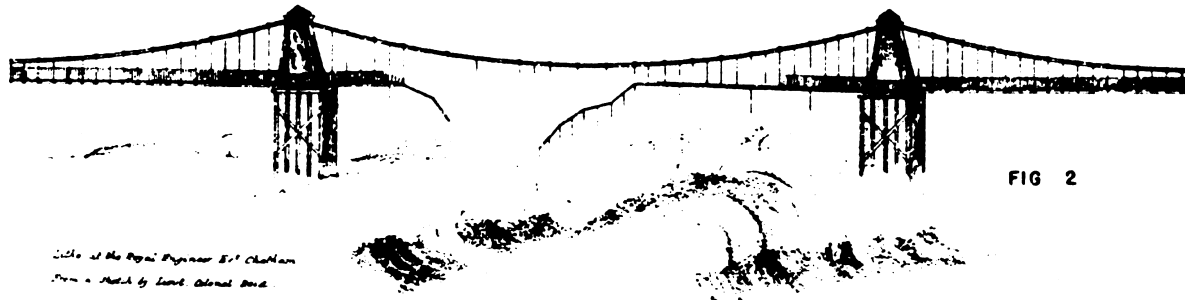
Figure 1.10 Failure of the Brighton Chain Pier, 1836.
