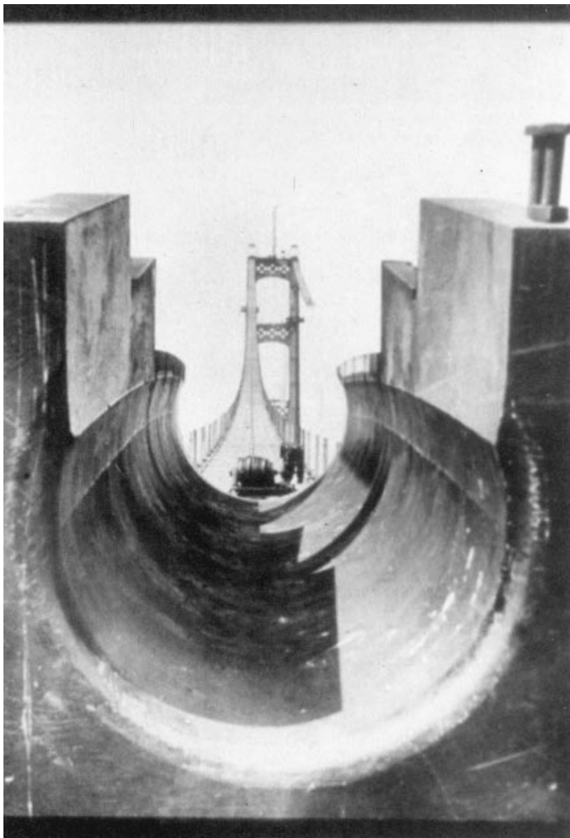
FIGURE 15.35 Pylon saddle.
